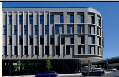
Hotel Cloud One, Prague 1 ■ Developer: Penta Real Estate ■ Facility management: Rilancio ■ Source: Klinker
