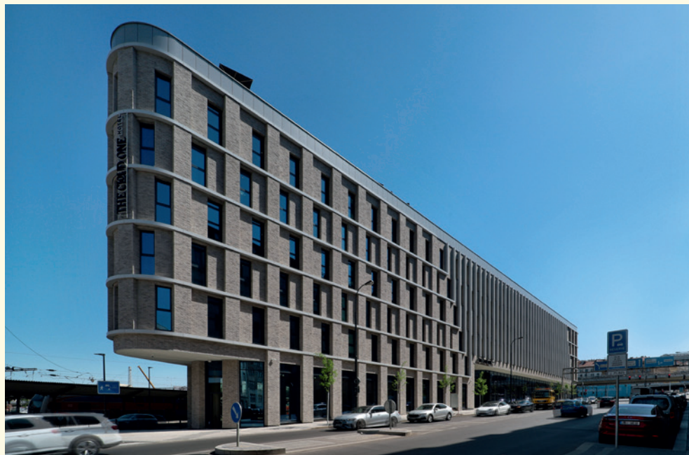
Hotel Cloud One, Prague 1 ■ Developer: Penta Real Estate ■ Facility management: Rilancio ■ Source: Klinker
