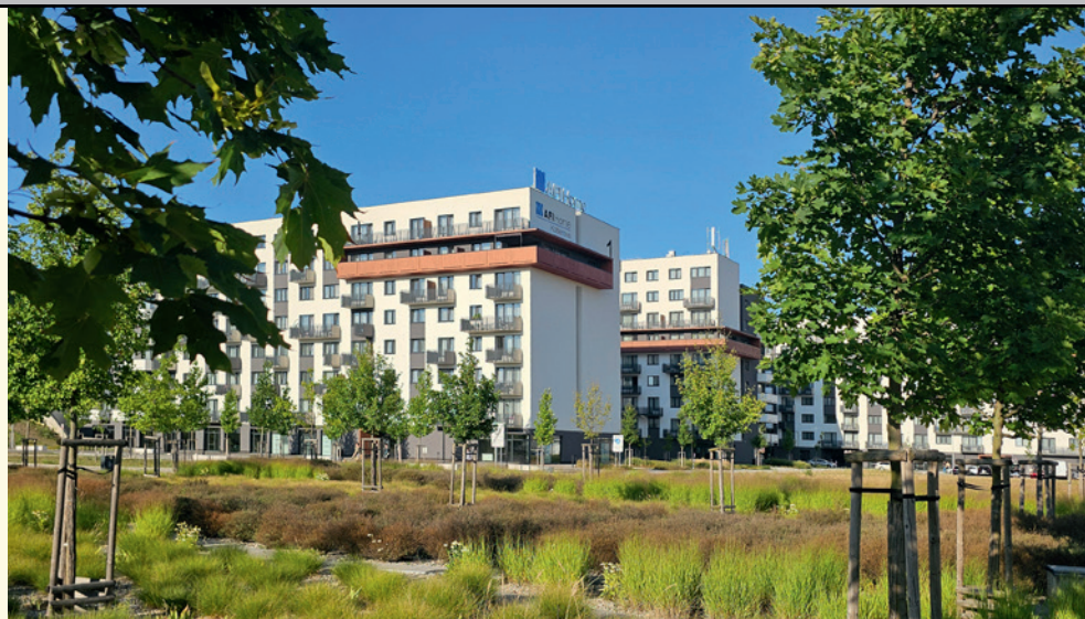
AFI Home Kolbenova, Prague 9 ■ Investor: AFI Europe ■ Facility management: Rilancio
