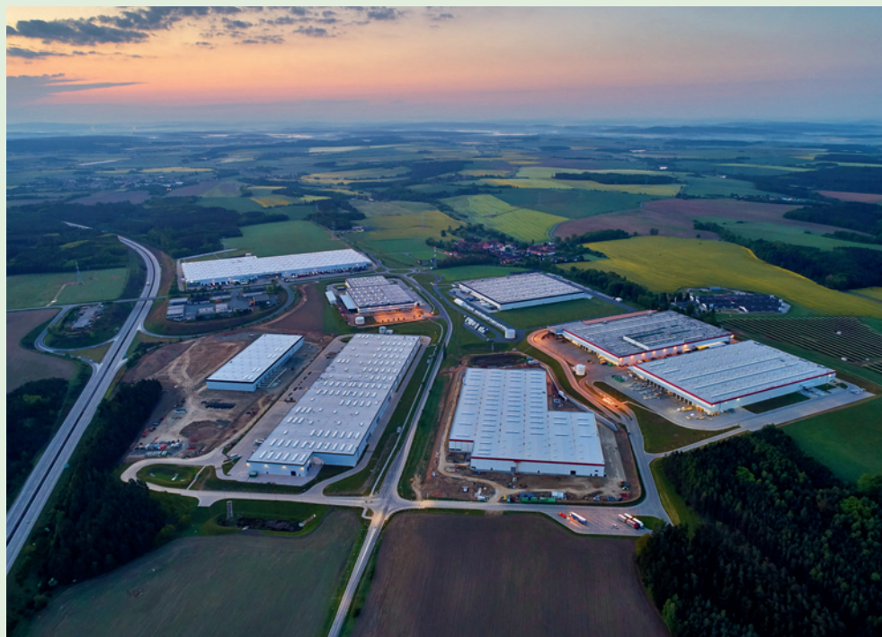
Panattoni Park Ostrov u Stříbra ■ Developer/Investor: Panattoni/Accolade ■ Technical facility management: Rilancio
