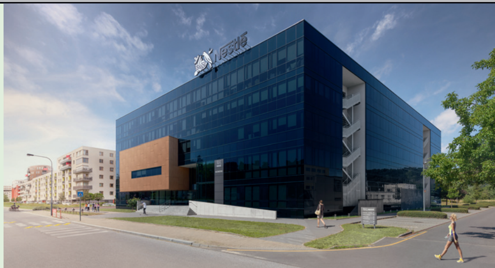
Mezi Vodami Office Building, Prague 4 – Modřany ■ Technical facility management: Rilancio
