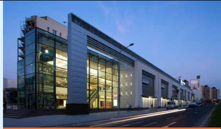
Central Most shopping centre ■ Technical FM: Rilancio
