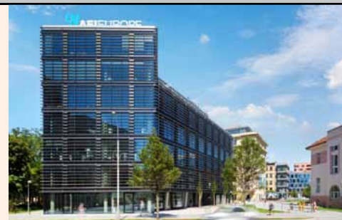
Classic 7 – phase III ■ Facility management: Rilancio
